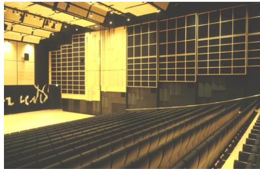
*Three view's of the hall with the absorbing side wall panels extracted (black squares).*
